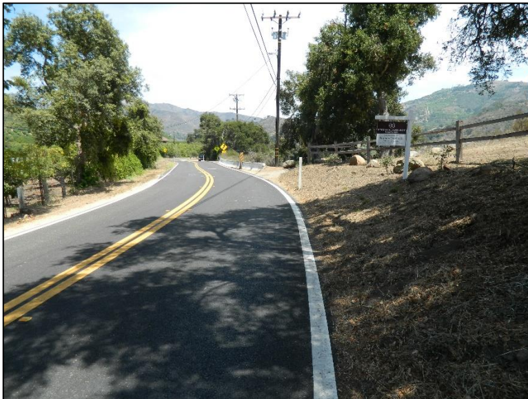
Photo 6 - HDD exit area on Casitas Pass Road (Highway 192) looking northeast, approximately El. 190. Layout pipe string area down Casitas Pass Road to photo foreground.
