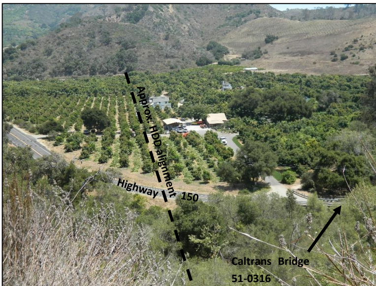
Photo 2 – View of HDD alignment looking down eastward from Casitas Pass Road (Highway 192) to the Abbott/Solis orchards.
