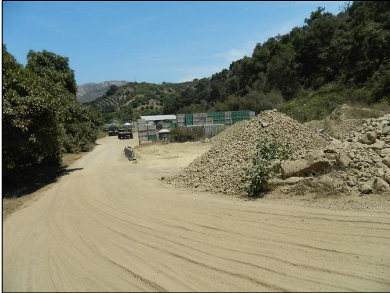
Photo 5 – HDD rig side entry area. Gravel piles to be removed (the gravel, cobbles and boulders stockpiled here are imported, not derived from the project alignment).
