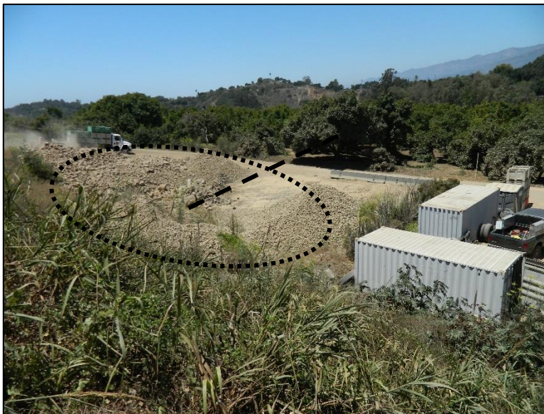
Photo 4 – HDD rig side entry area, approximately El. 180.
