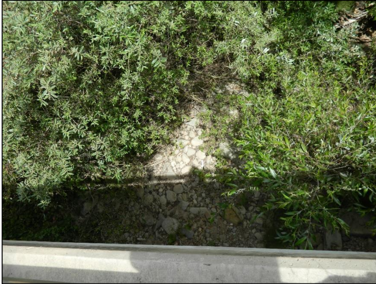
Photo 9 – View of cobbles and boulders in the creek bed of Rincon Creek taken from Caltrans Bridge 51-0316.
