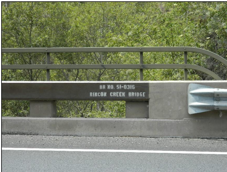
Photo 8 – Caltrans Bridge 51-0316 over Rincon Creek close to the HDD alignment, approx. 100 feet south of the HDD alignment.
