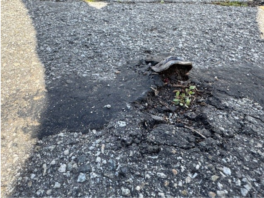
Bolt and washer above grade
