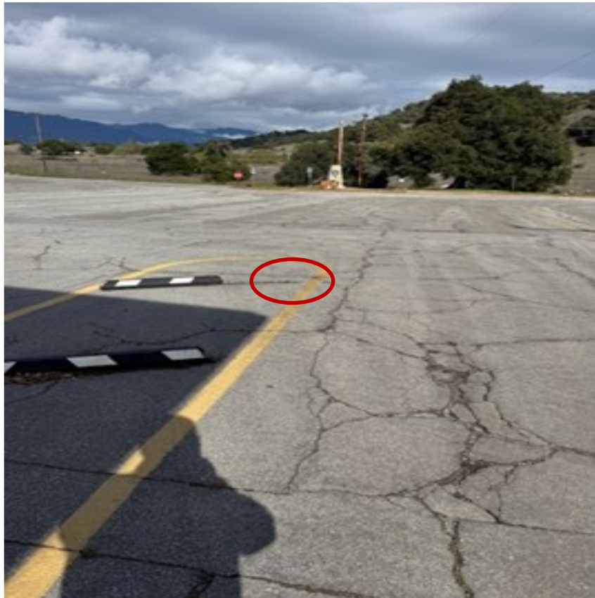
View Looking Past Exit-Santa Ana Road Ahead
