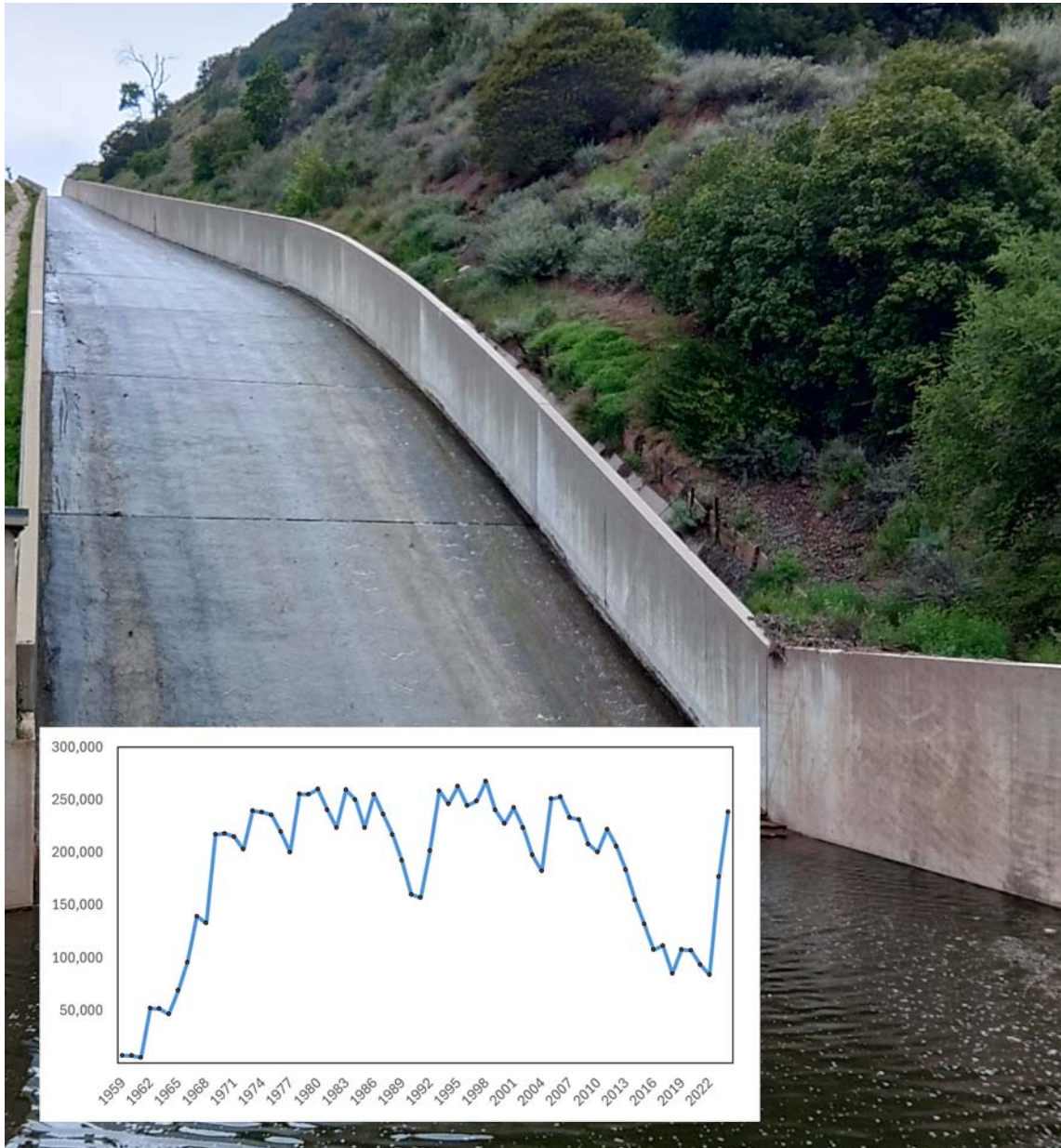
Photo of the Lake Casitas Dam spillway, which spilled for the first time since 1998, and graph of historic water storage of Lake Casitas (1959-2024).
